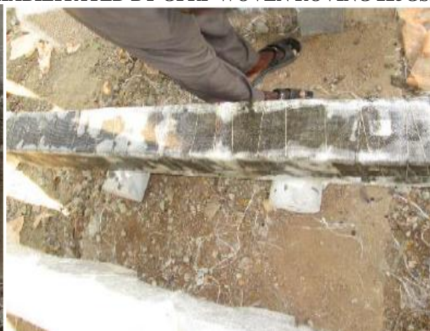
FIG 9AFTER APPLYING RESIN FOR BONDING
