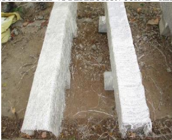
FIG 8 GFRP WRAPPED BEAM
