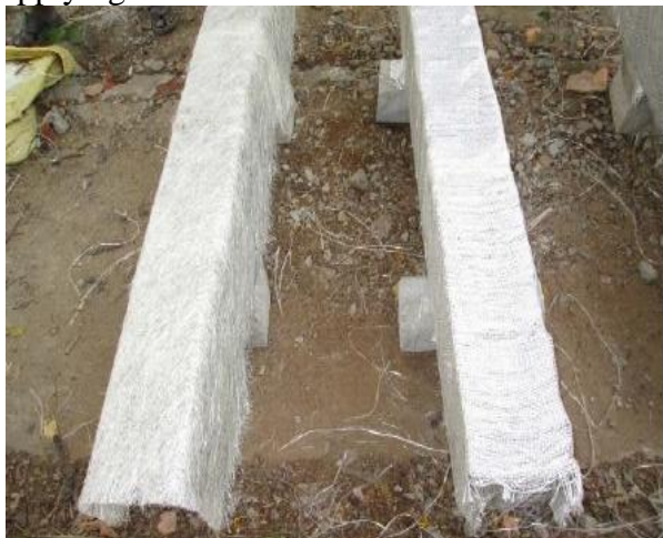
FIG 13 GFRP CSM 300 GSM WRAPPED BEAM
