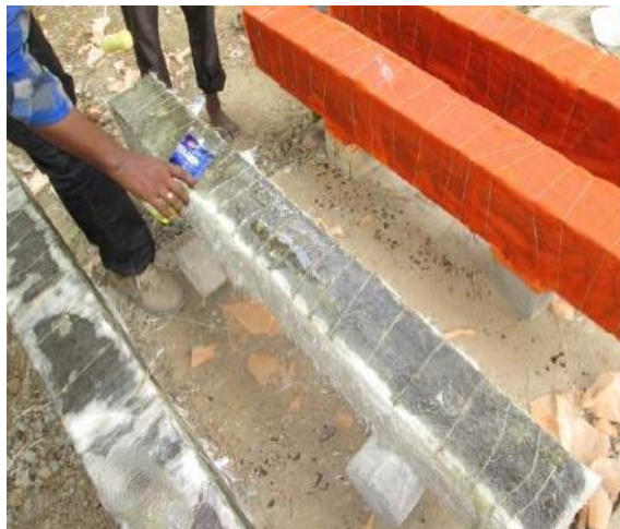
FIG 14 AFTER APPLYING RESIN FOR BONDING
