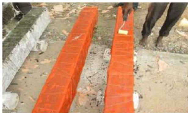
FIG19AFTER APPLYING RESIN FOR BONDING
