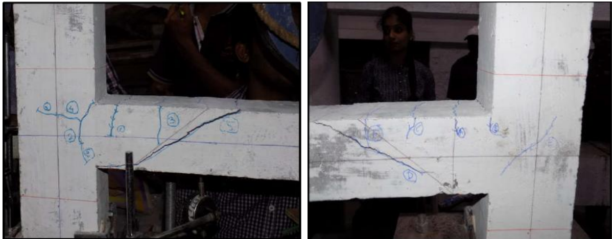
(a) CRACK PATTERN ON FACE A
