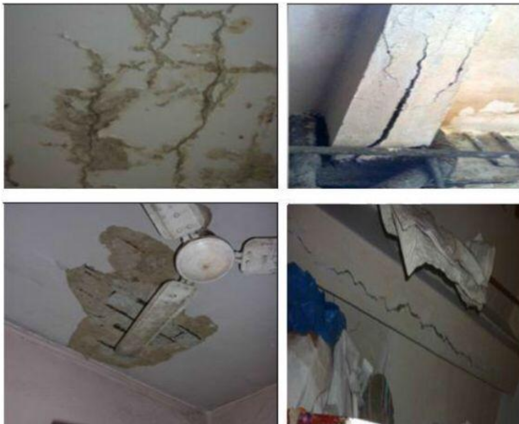
Fig. 2 Actual Photographs of Building No.4, Labor Camp, Matunga road, Mumbai Date: 2-2-16
